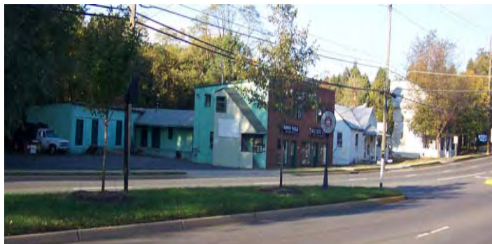
SW view of the Fairfax Depot area along s. side of Main St. (l to r) Fairfax Feed & Supply Store (c. 1925), Mill Managers House (1904), E.B. Rector House (1907).
