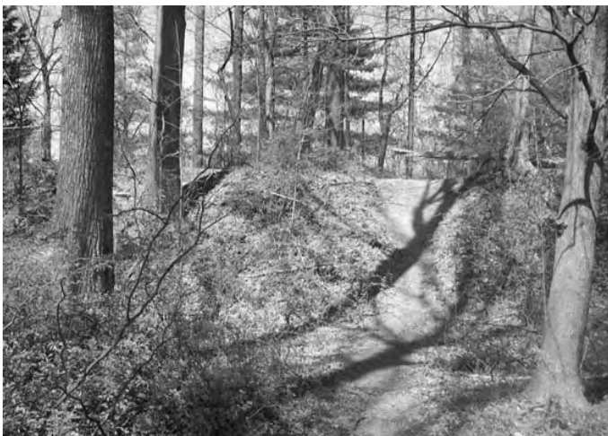
A "cut" in the line of the Unfinished Manassas Gap Railroad. Higginbotham Property, City of Fairfax. Photo credit: Page Johnson
