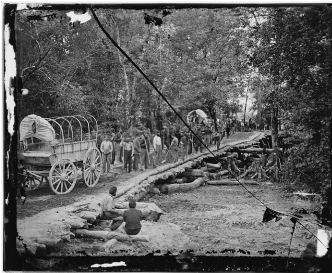
Union soldiers constructing a corduroy road and bridge across the Chickahominy River, near Richmond, VA, 1862.
