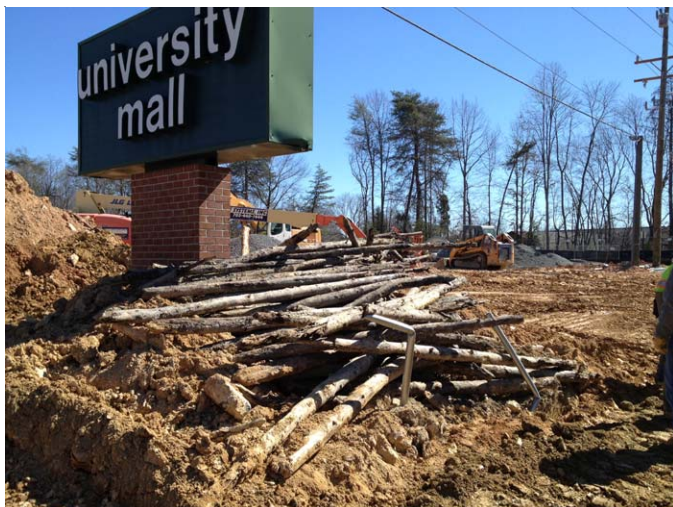
Excavated logs from the corduroy road awaiting recovery. Photo credit: Chris Martin
