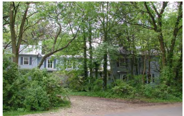
Roberts/Chichester House from Stratford Avenue. Earliest portion of house on right.
