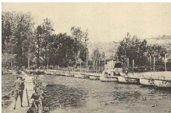
Pontoon bridge across the Marne River, near Chateau Thierry. Built by U.S. Engineers, July 1918.
